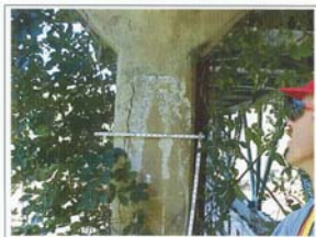
Delamination and crack in column "B" of pier no. 3
