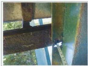
Hole in top flange of LBR-LBL, truss no. 3 at pier no. 3
